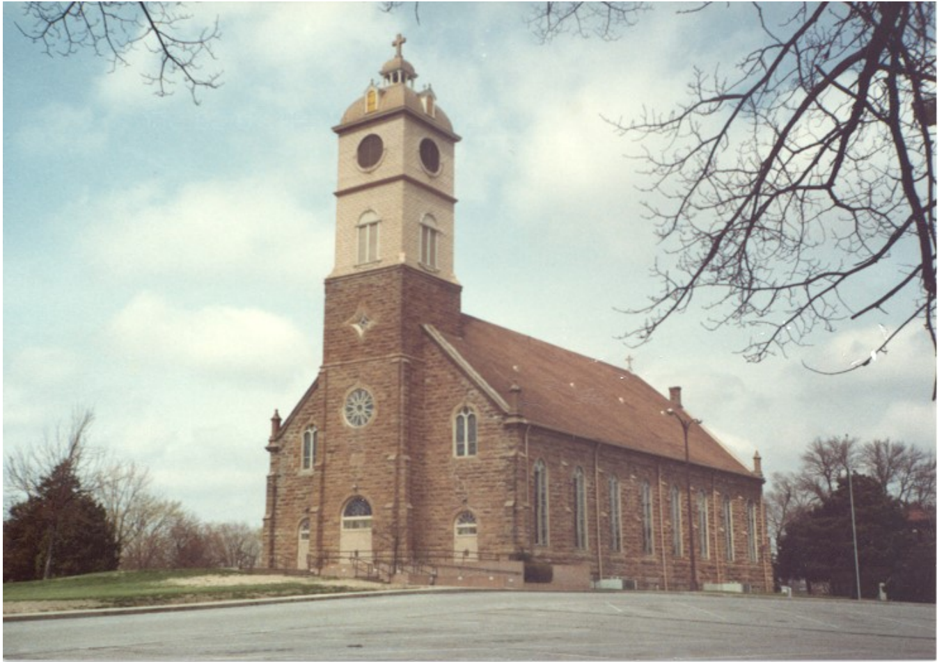
The exterior of St. Francis de Hieronymo Church, St. Paul, Kansas.
